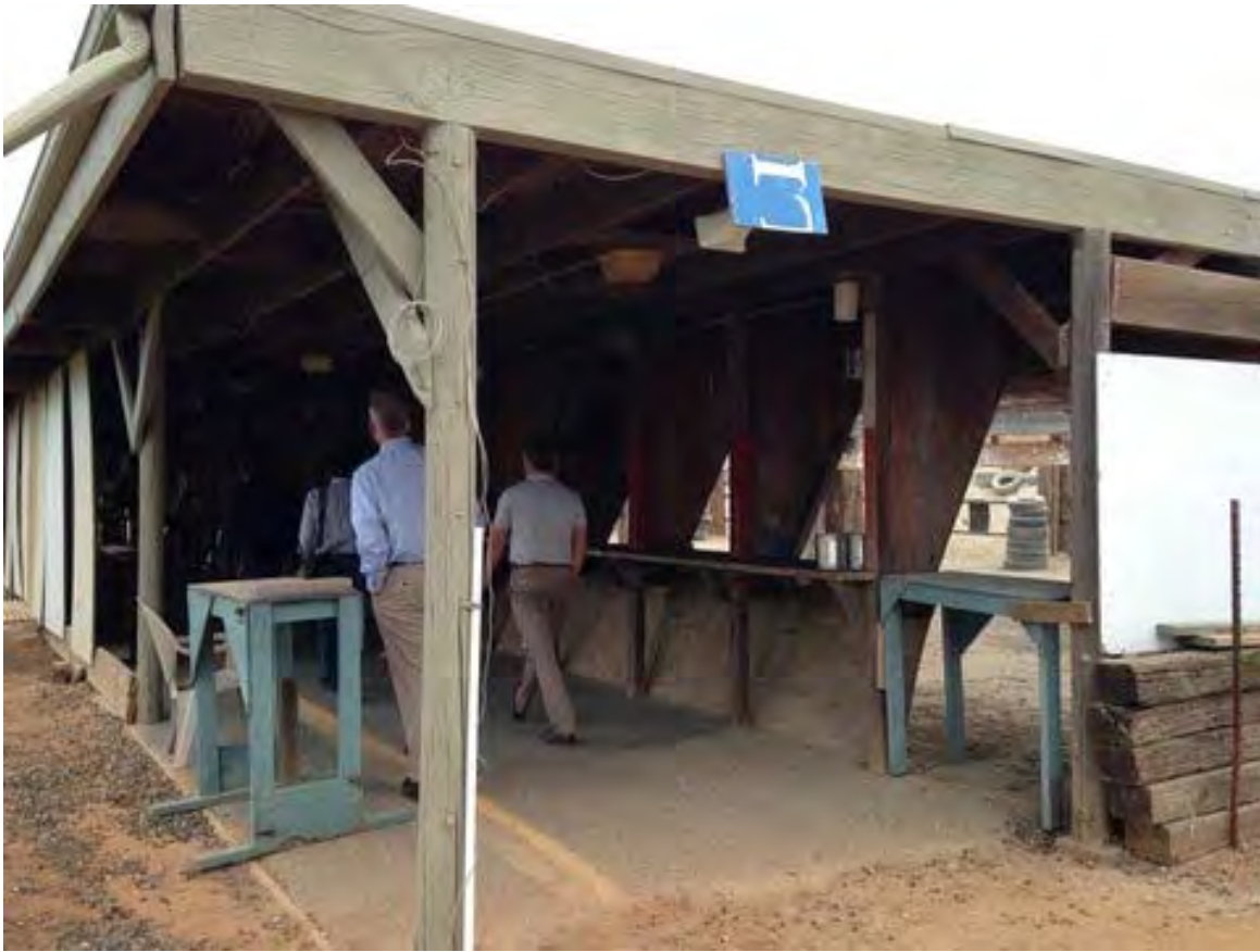
The facility lacks an accessible entrance, accessible pathway, or accessible shooting stalls.
