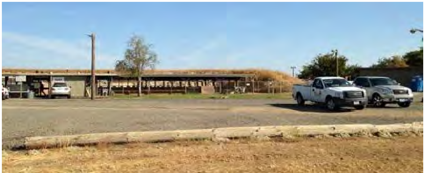
The facility lacks accessible parking and an accessible restroom.
