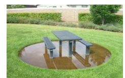
Figure 181 Drainage issues
