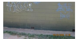
Figure 5 – Damage to Bleachers
