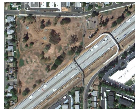
Figure 225 – Aerial Photo of the park under construction
