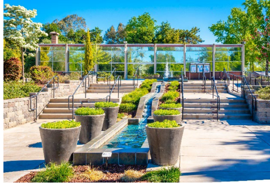
Hagan Community Center - Building 1
