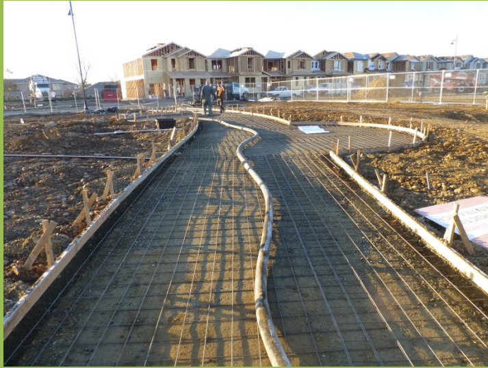
Concrete formwork begins in December
